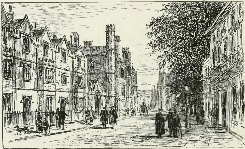
Corpus Buildings, Cambridge
